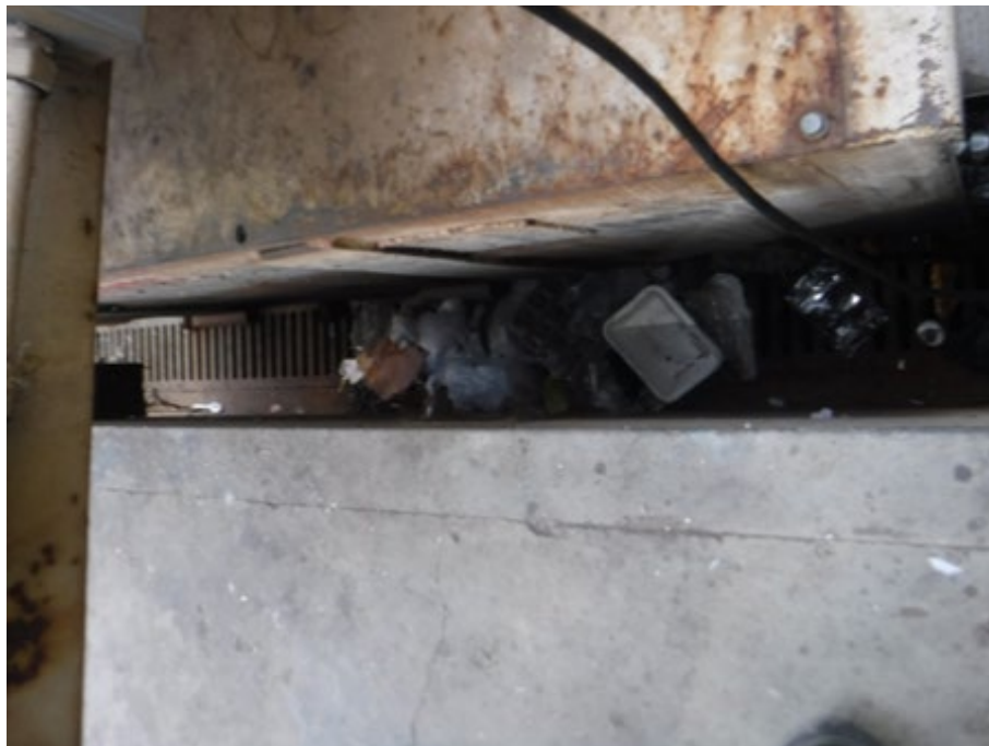
SD_743872 – Vista (Kitchen dumpster ground area)
