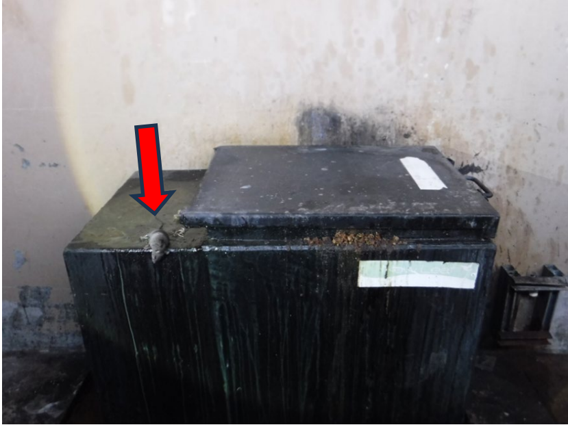
SD_743887 – Vista (Kitchen loading dock)
