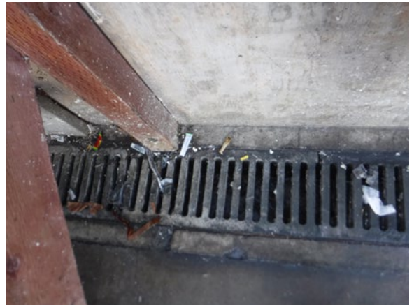
SD_743877 – Vista (Kitchen loading dock)
