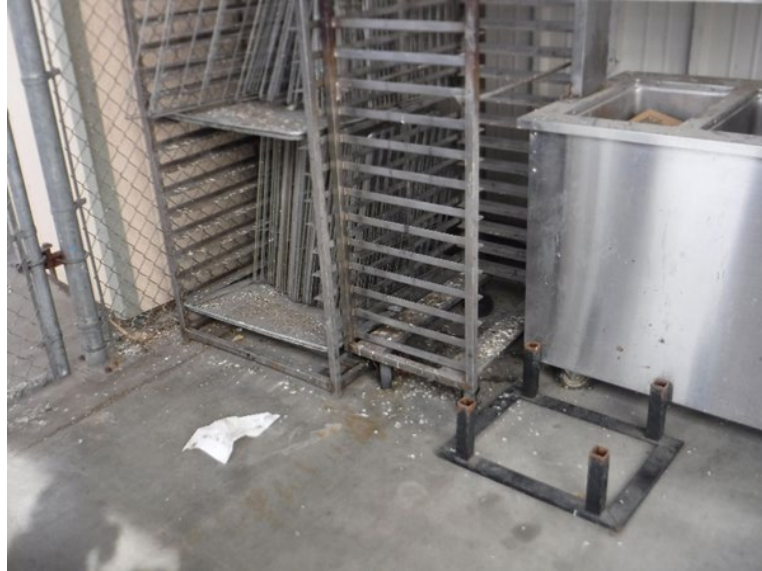
SD_745518 – East Mesa (Loading dock)
