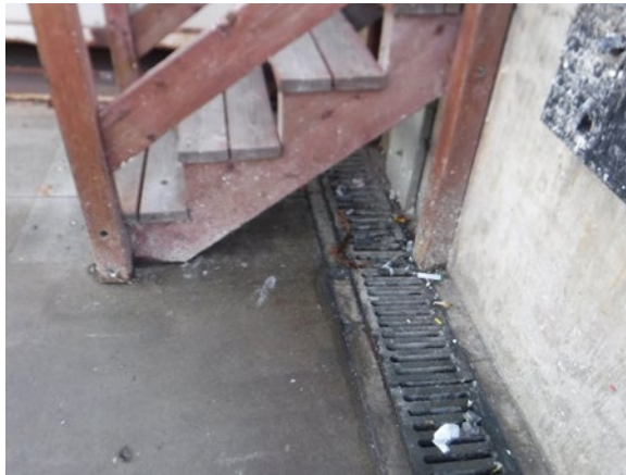
SD_743884 – Vista (Kitchen loading dock)
