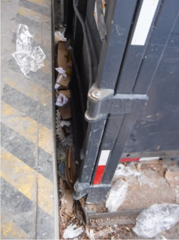
SD_745511 – East Mesa Kitchen (Dumpster area)
