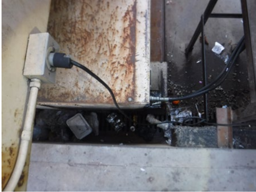
SD_743873 – Vista (Kitchen dumpster ground area)
