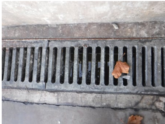
SD_743880 – Vista (Kitchen loading dock)
